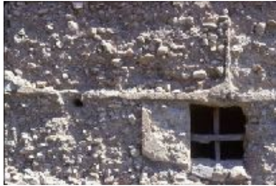
WALL BY ESTABILIZED EARTH
