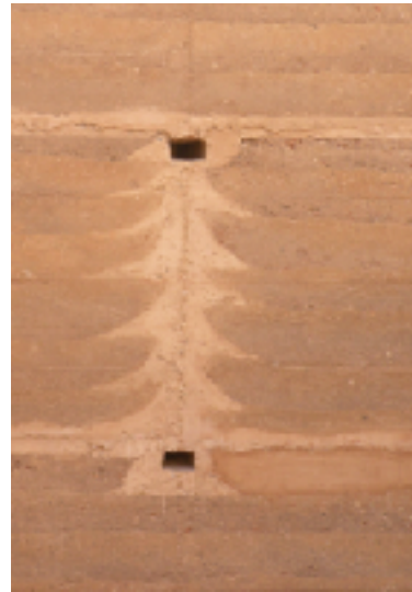
WALL BY ESTABILIZED EARTH
